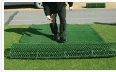
2 Spread the mat along walking direction
