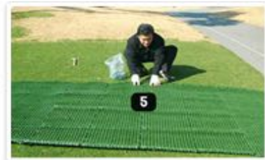
9 Pins are fixed on each side of the mat.
