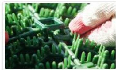
12 Pegs should be well inserted inside the four holes in the middle of the mat.
