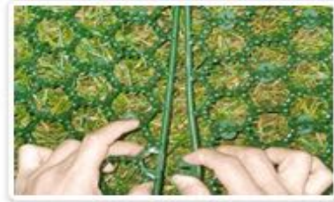
3 Reassemble the mat if it is not placed along walking direction.
