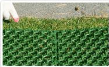
4 Distance 5cm to 10cm from the road to make pins easy to fix, (No grass damage)
