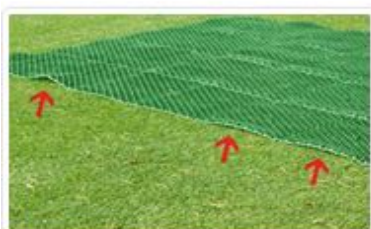
13 Additional pins are fixed if any sides of the mat are lifted.
