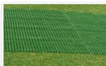
14 Our mat is completely installed.
